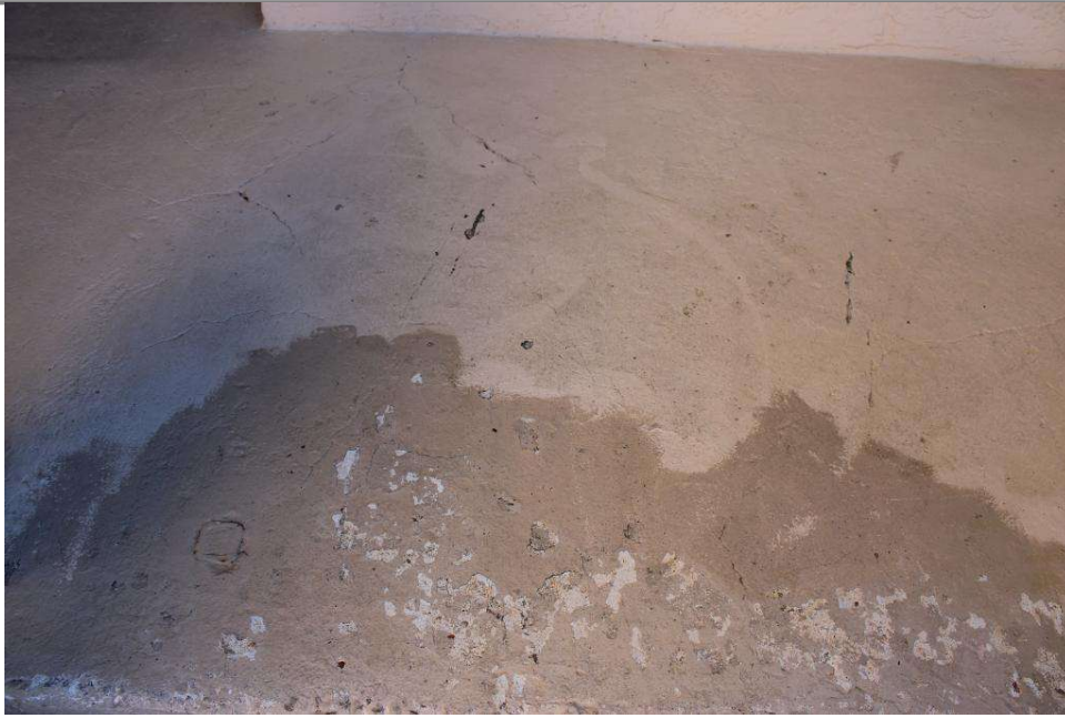
Exterior Building paint
