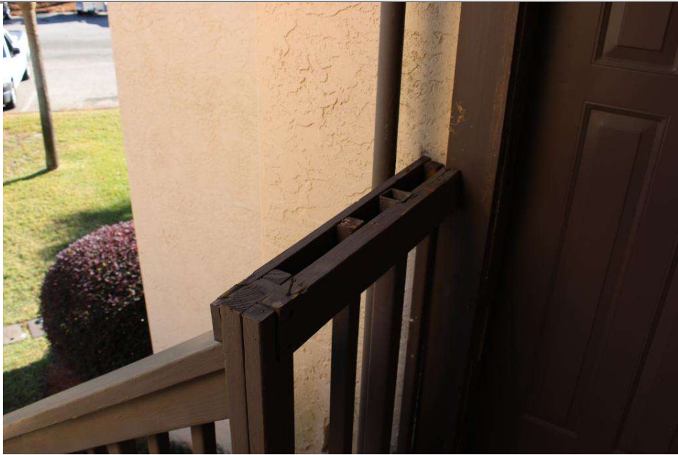
Guardrails Repairs (Front and Back of the Buildings)
