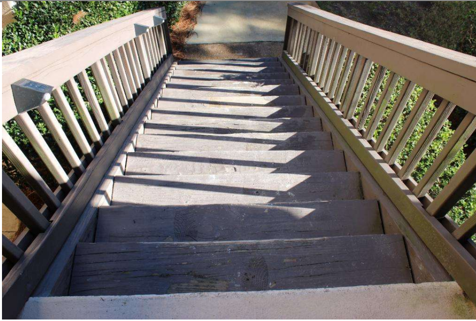
Exterior Building paint
