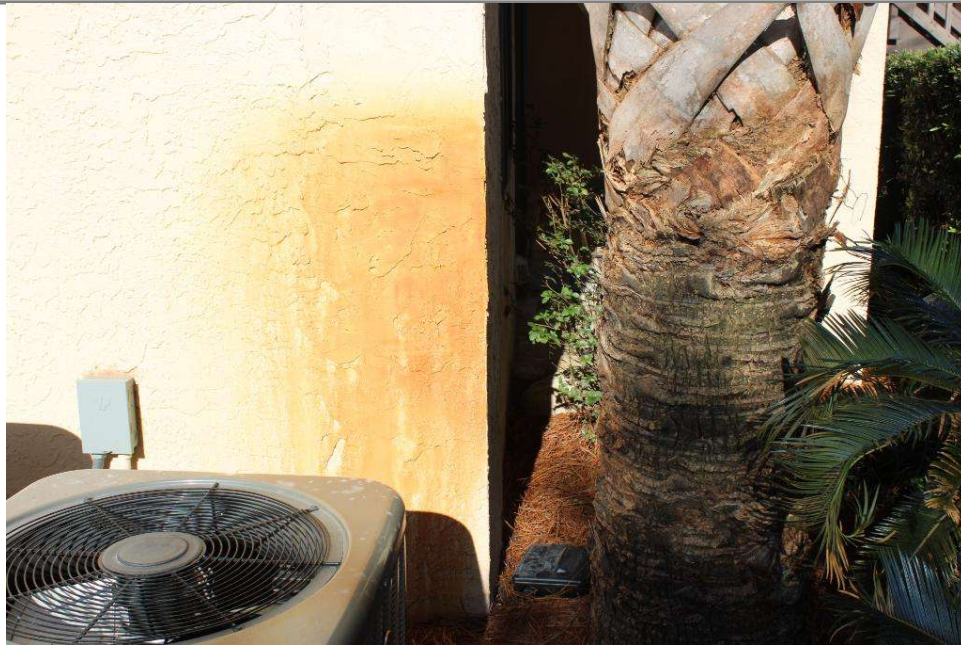
Exterior Building paint
