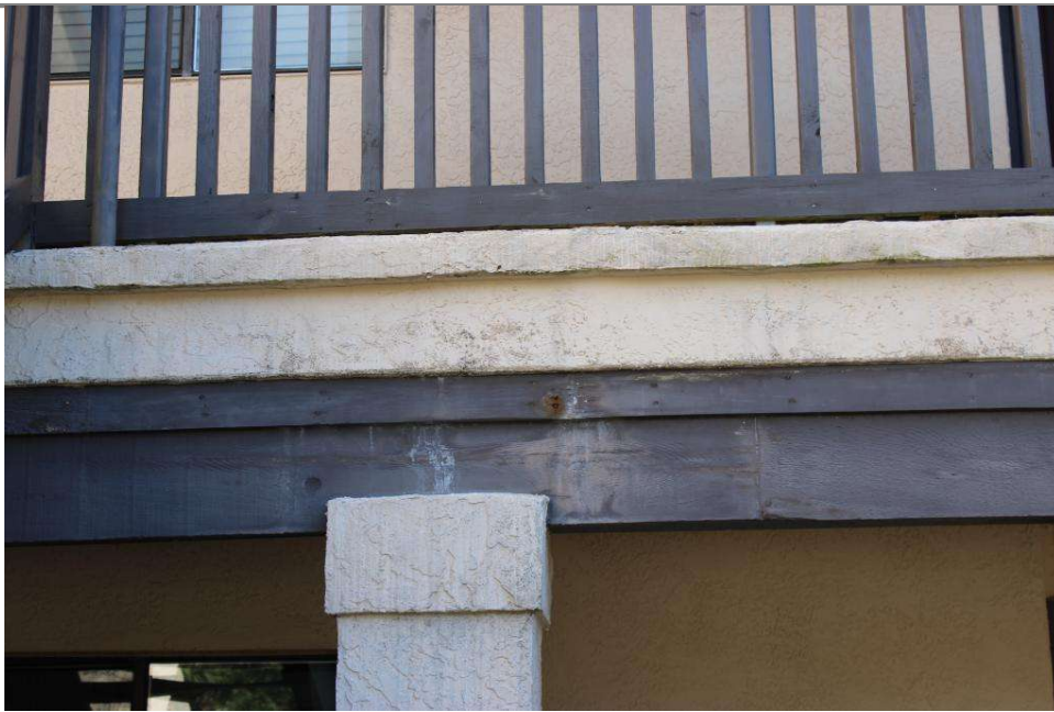
Exterior Building paint
